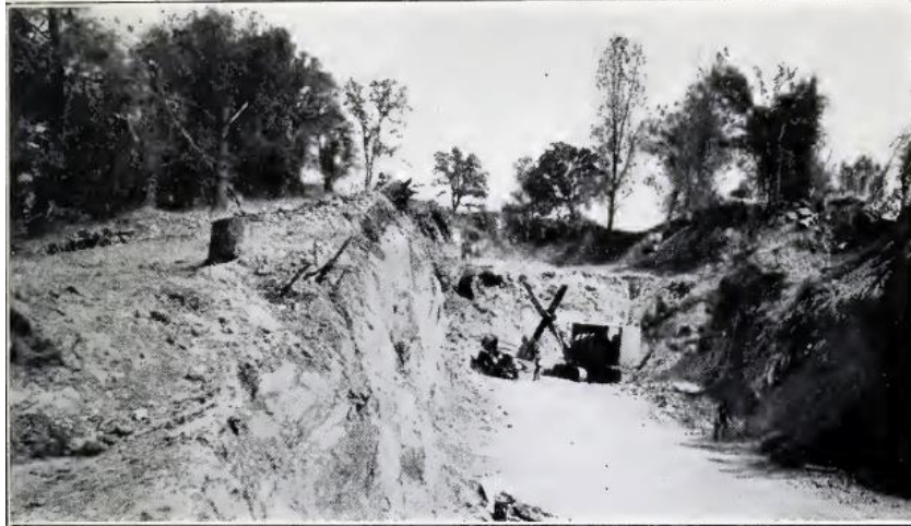
Open-pit mining of gold-bearing gossan ore at Dairy Farm Mine, 1935.
